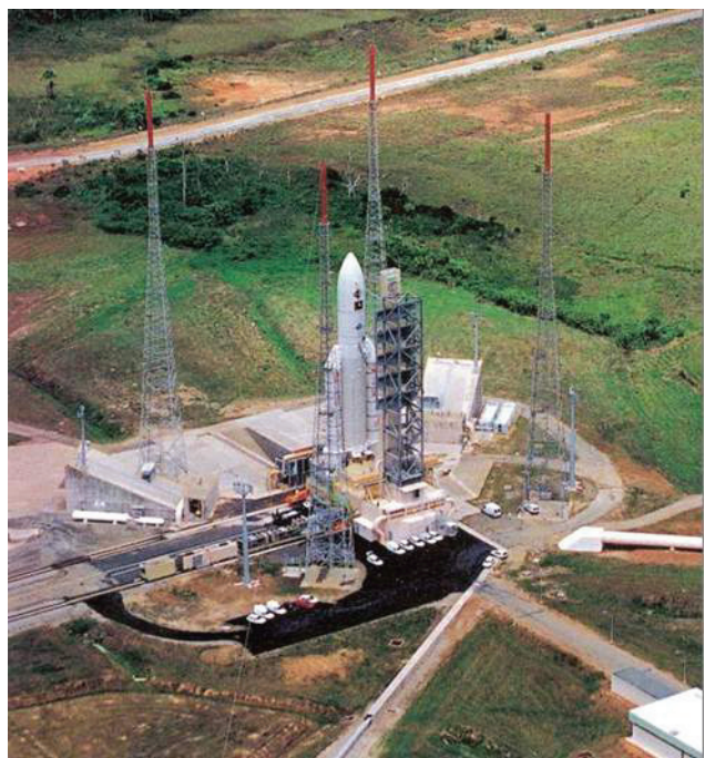
Figure 2 – Ground launch complex (appearance) [ https://www.flickr.com/groups/ares/pool ]
