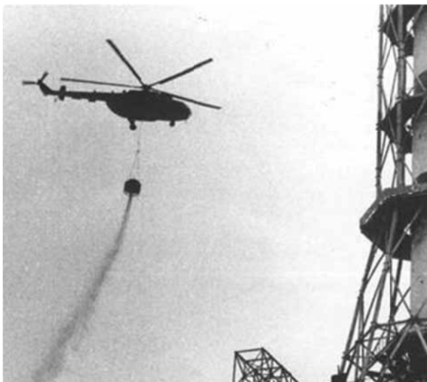
Figure 2. Helicopter sprays dust suppression reagents [3]
