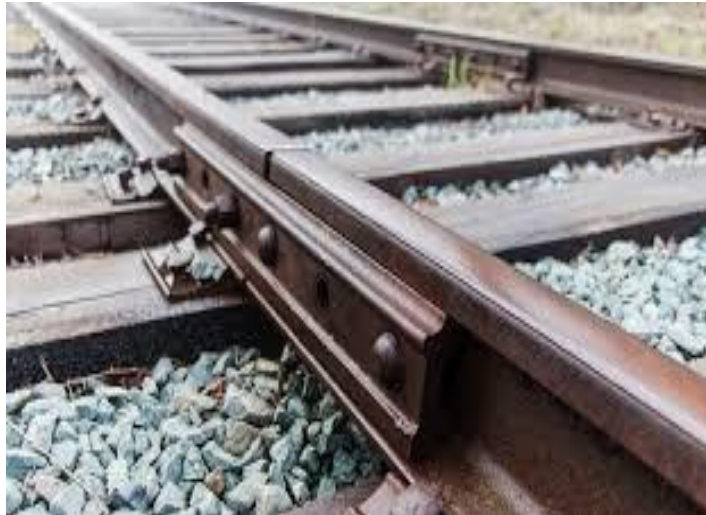
Figure 2.1. The railway track
